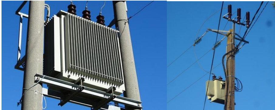
Figure 3-1 Dual pole transformer in Wallonia (BE)(Left) (source: www.gregor.be ) and single pole in France (right) (source: https://fr.wikipedia.org/wiki/Poste_%C3%A9lectrique )
