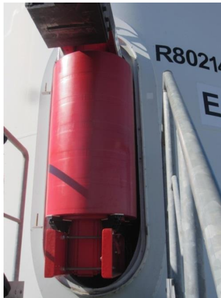
Figure 1-7 dry type transformer installed in wind turbine tower with dimensional constraints (Source: EDF EN (Energies Nouvelles) (2016))
