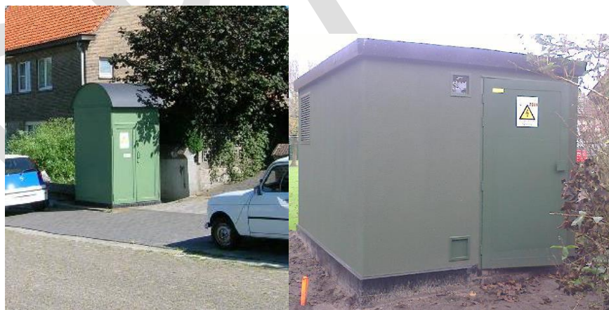
Figure 1-6 metal substation max. 250 kVA(left) and standard concrete prefabricated substation max. 630 kVA (right) with dimensional and weight constraints (Source: Synegrid BE (2016))
