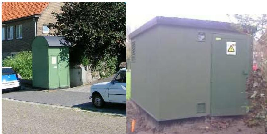
*Figure 1-7 Metal substation max. 250 kVA (left) and standard concrete prefabricated substation max. 630 kVA (right) with dimensional and weight constraints (Source: Synegrid BE, 2016)*
