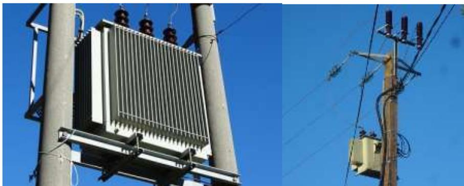
Figure 3-1 Dual pole transformer in Wallonia (BE)(Left) (source: [www.gregor.be](http://www.gregor.be)) and single pole in France (right) (source: [https://fr.wikipedia.org/wiki/Poste\\_%C3%A9lectrique](https://fr.wikipedia.org/wiki/Poste_%C3%A9lectrique))
