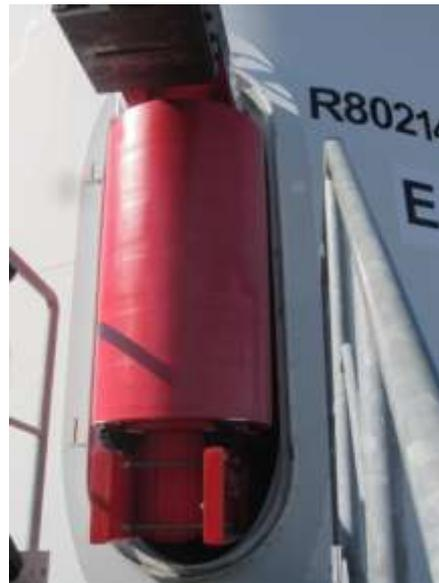
*Figure 1-8 Dry type transformer installed in wind turbine tower with dimensional constraints (Source: EDF EN (Energies Nouvelles), 2016)*
