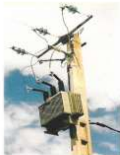
Mounted on 1 pole 350 000 units 50-160 kVA Max. 550 kg
