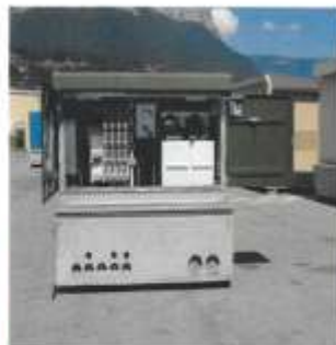
Semi-rural substation 130 000 units Max. 250 kVA Max. 1500 kg Floor space < 2,5 m 2 Height < 1,5 m
